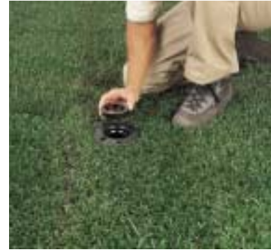
3. Thread on adapter cap and securely tighten.
