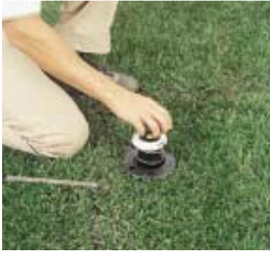
1. Remove internal assembly of existing sprinkler.
