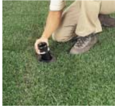
2. Insert the retrofit adapter sleeve. Press the snap ring into position to secure adapter.
