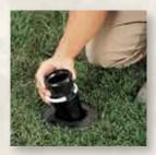
2. Insert the retrofit adapter sleeve. Press the snap ring into position to secure adapter.
