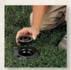
3. Thread on adapter cap and securely tighten.
