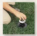
1. Remove internal assembly of existing sprinkler.
