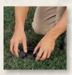
5. Snap the retaining ring in place.
