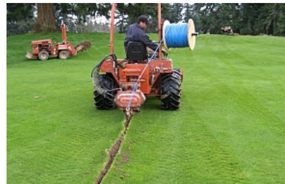
CABLE NEEDED FOR A TWO-WIRE DECODER SYSTEM
